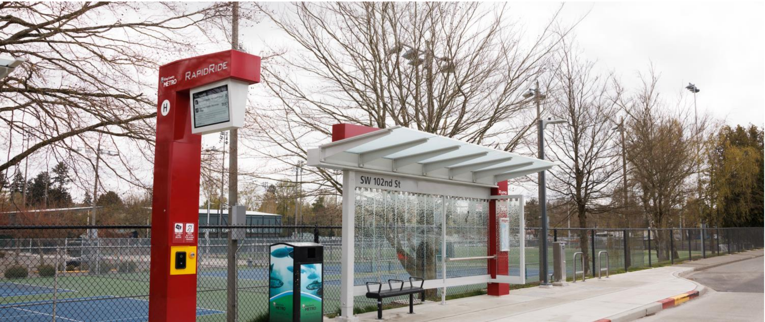
Example of a Large Station
